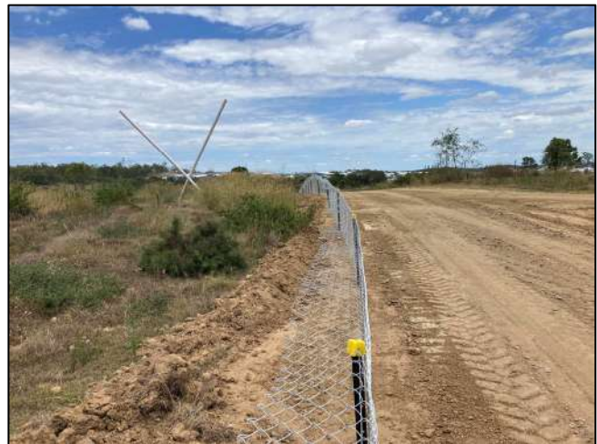
Photo Set 1: Temporary tree protection and floppy top fauna fencing.
