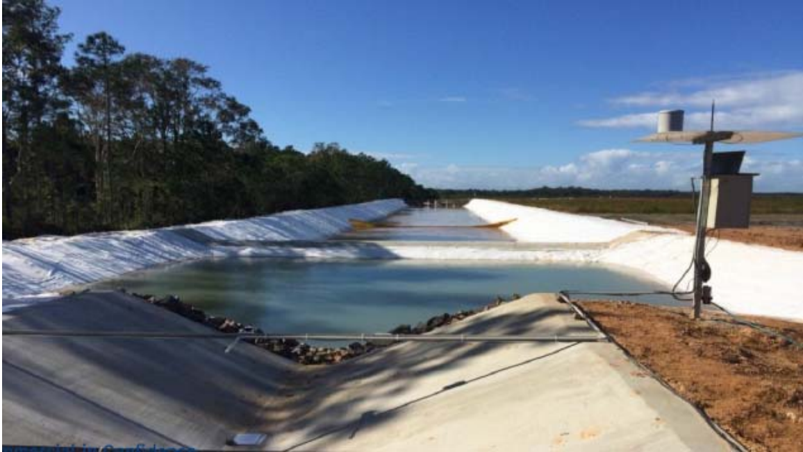
Figure 6: High Efficiency Sediment Basin Installed as Part of Precinct 1 Works
