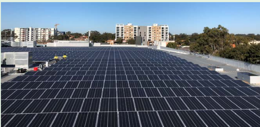
Solar panels now extend across the roof of Stockland Merrylands (NSW), scheduled for commissioning in early FY19.
