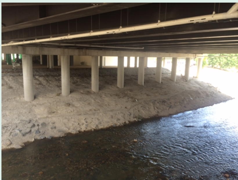
Moore's Creek flowing under a section of our Rockhampton shopping centre showing reinforcing to the structural footings.
