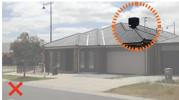
Non compliant evaporative cooler unit located at front of roof
