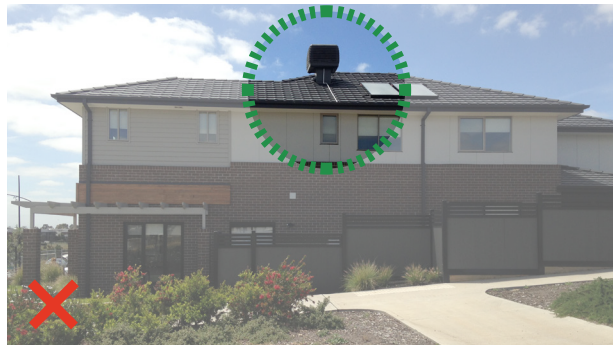
Non compliant evaporative cooler unit above roof ridgeline
