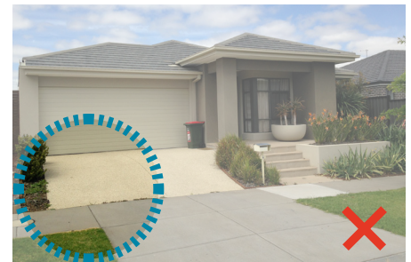
Driveway does not align with crossover
