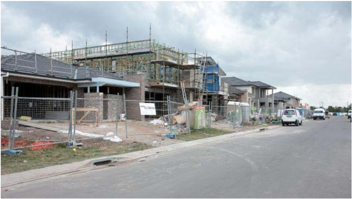
📷 Marsden Park is in the booming northwest corridor.
