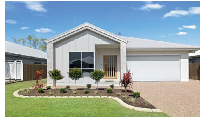
7. Keir Constructions Bella – Scandinavian Facade
