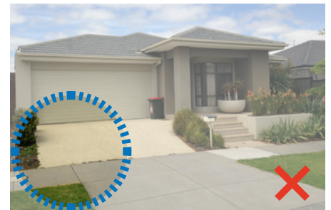
Driveway does not align with crossover
