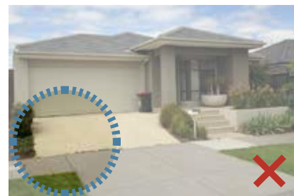
Driveway does not align with crossover
