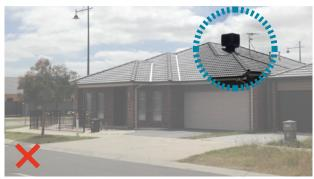
Non compliant evaporative cooler unit located at front of roof
