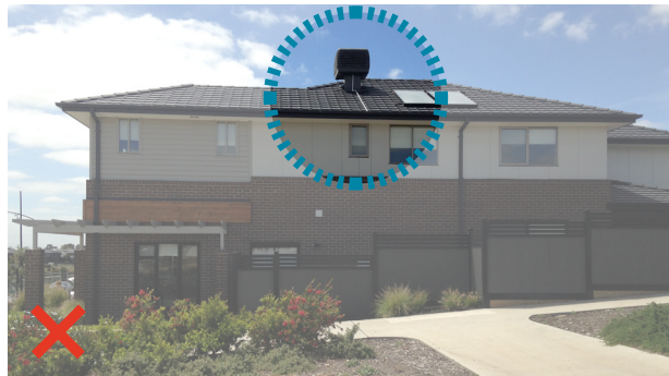
Non compliant evaporative cooler unit above roof ridgeline
