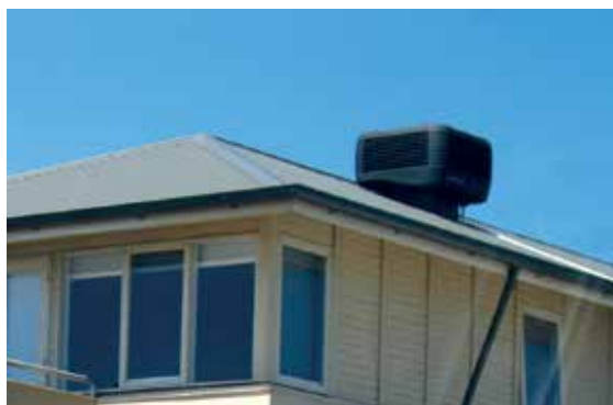
FIGURE 16 LOW PROFILE ROOF MOUNTED EVAPORATIVE COOLING UNIT
